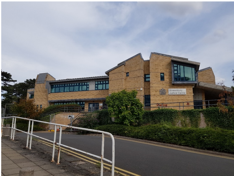
Figure 13. Shrewsbury Justice Centre, 1992 with additions. 2022. Credit: Wendy Horton/VCH Shropshire
