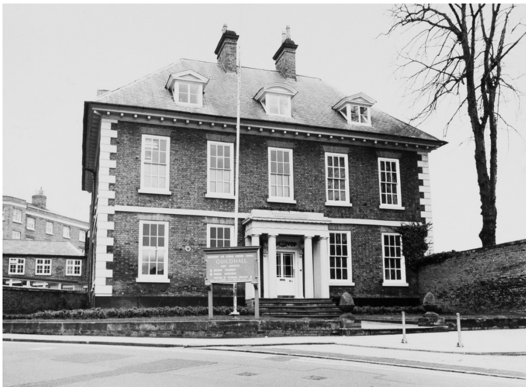
Figure 9. Newport House: The Guildhall, c. 1980. Credit: SA, PHS/13/D/3/62. Copyright: Shropshire Magazine
