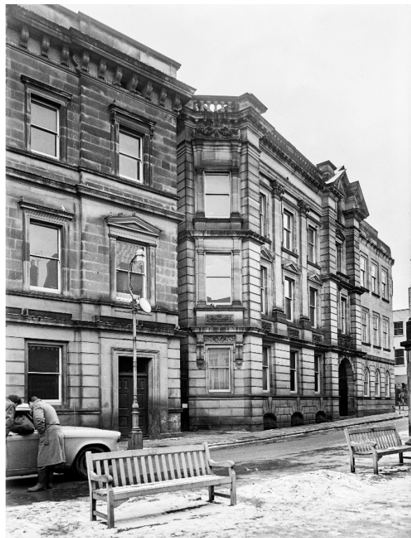
Figure 7. The Shirehall, including extensions of 1906 and 1938. Credit: AA63/02182: RBEP 5126_025 (GB Mason, 1963). © English Heritage Archive
